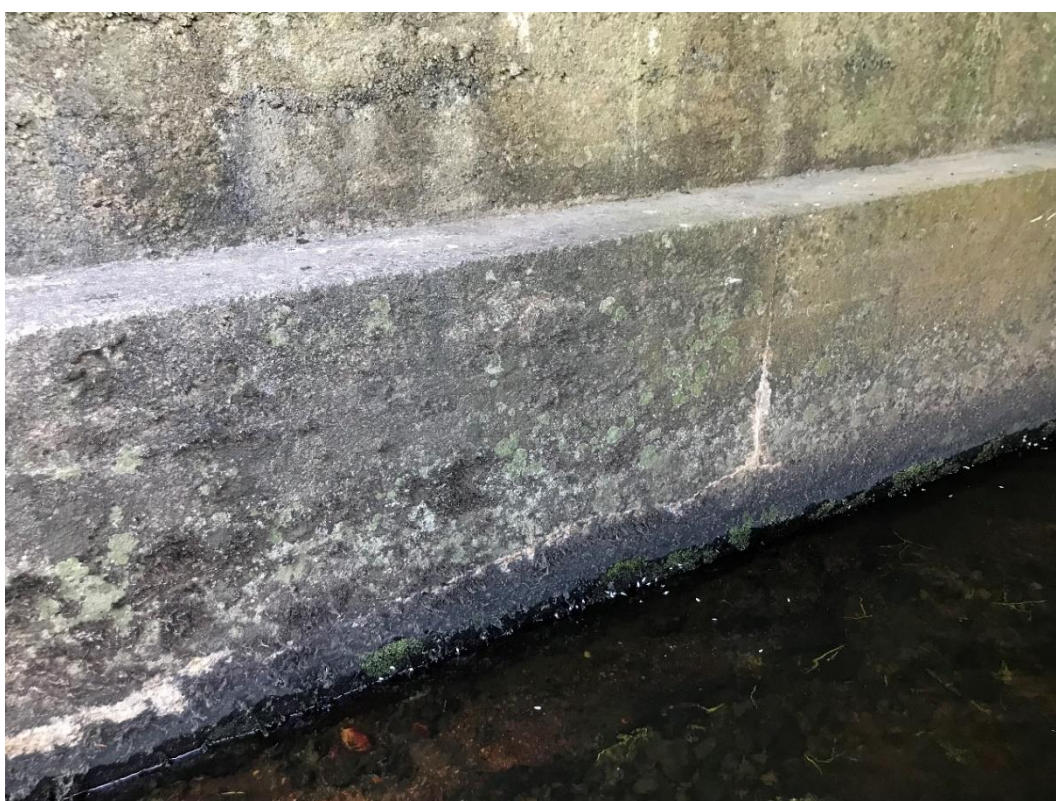
Figure H-14 – View of the cracking to the north face of the pier
