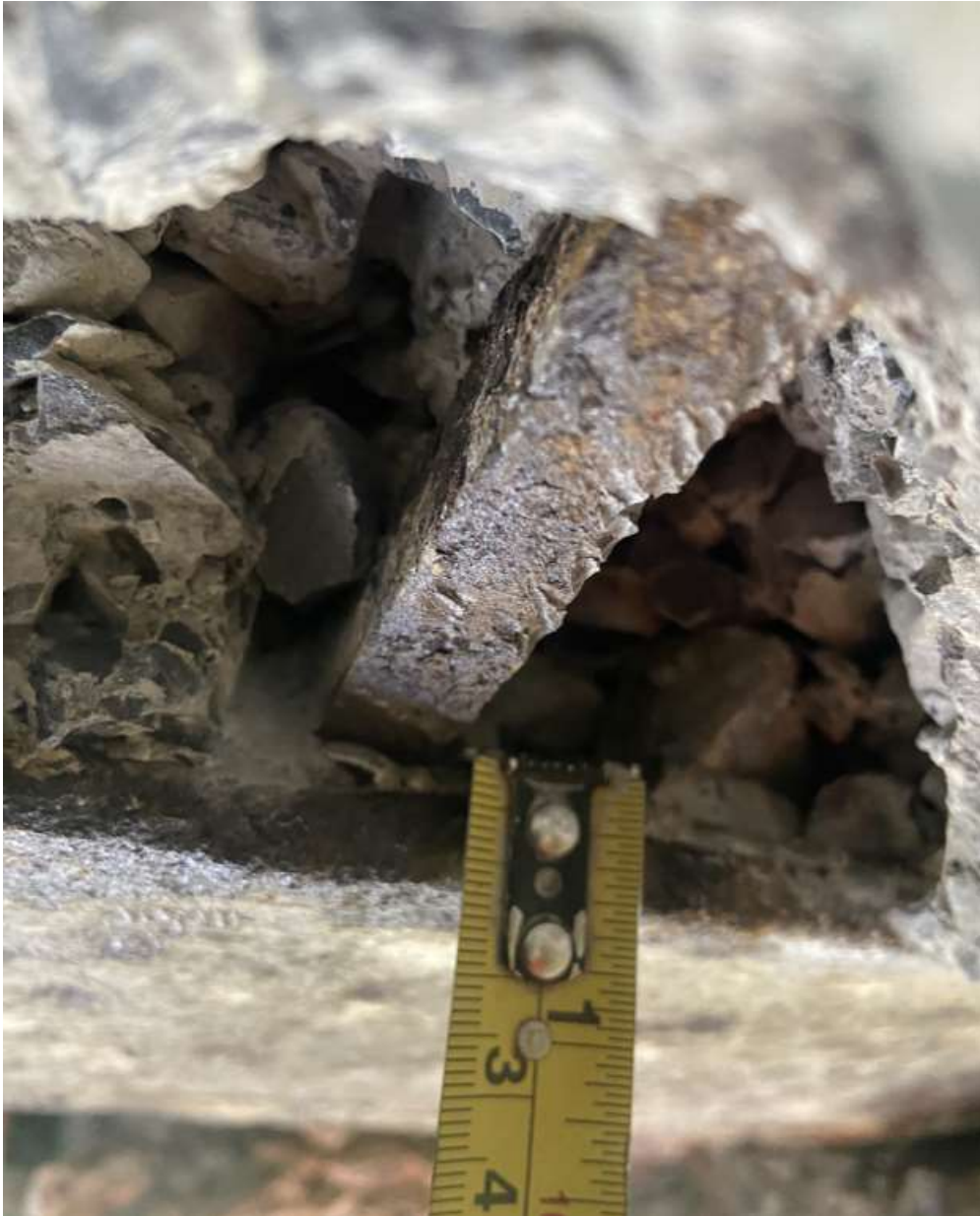
Figure 40: Longitudinal bottom flange thickness
