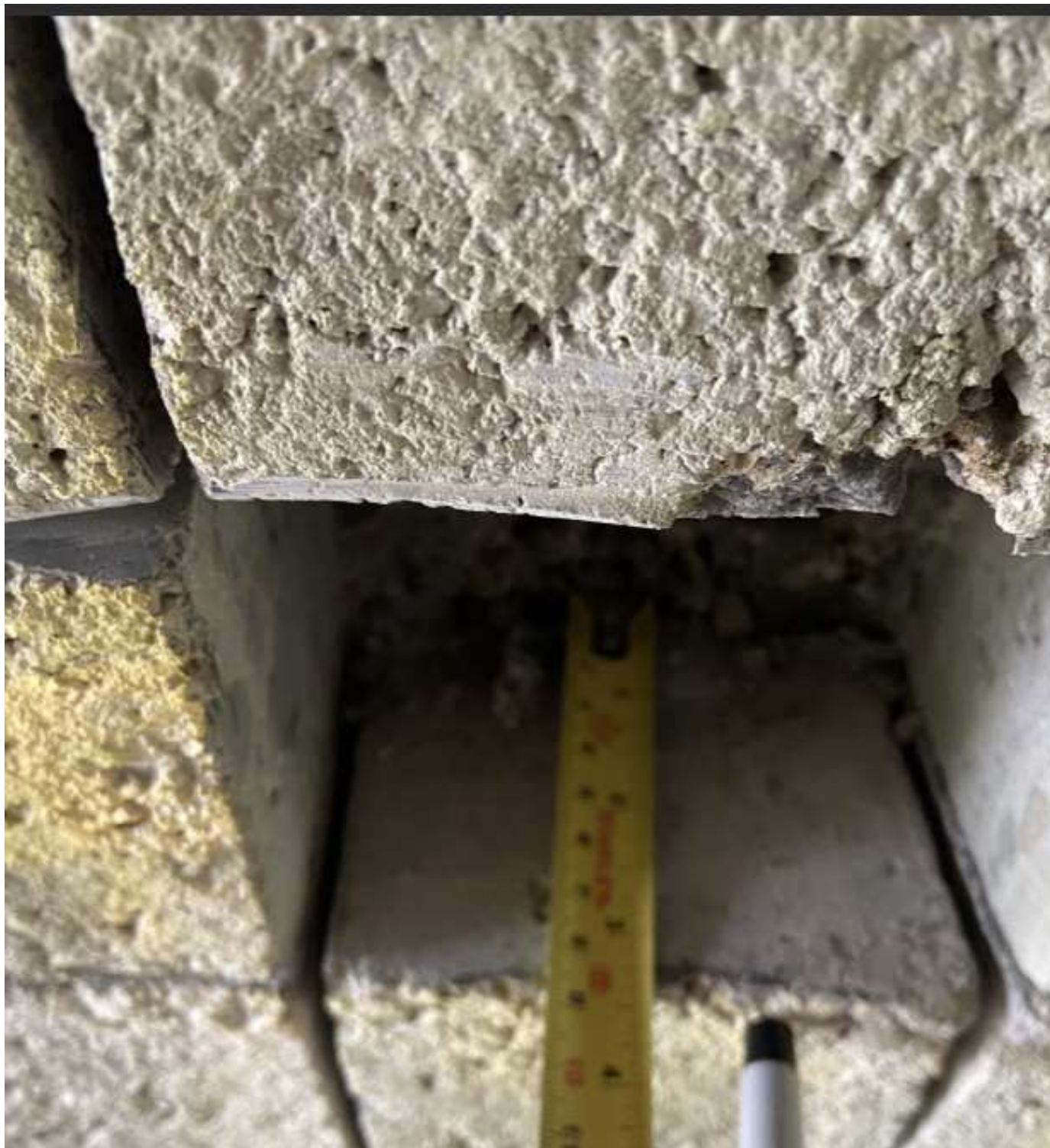
Figure 49: TA6 carbonation sample depth into pier
