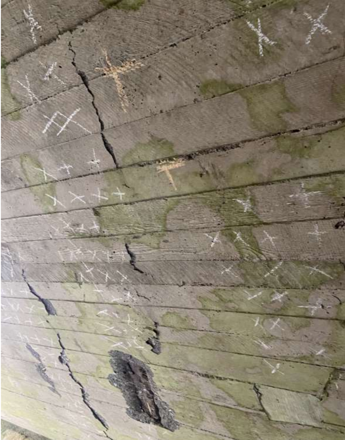
Figure 29: Further delamination on south arch
