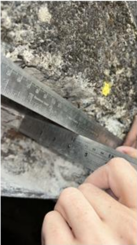
Area 3 - Top side flange 105mm cover side
