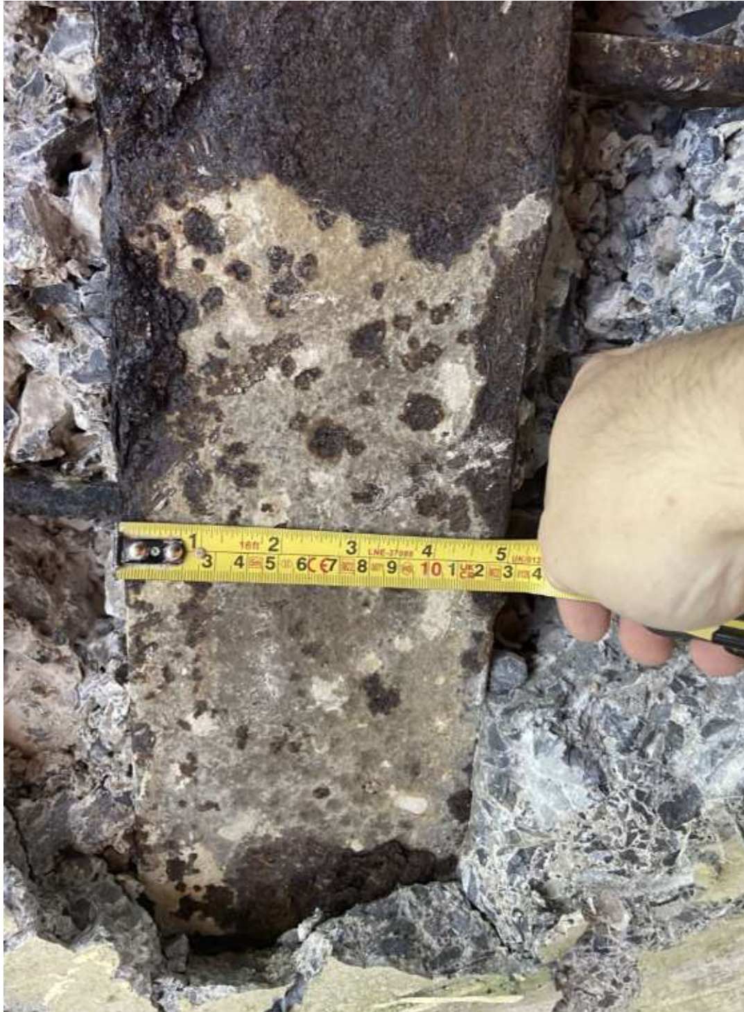
Figure 42: 125mm wide bottom flange of internal beam
