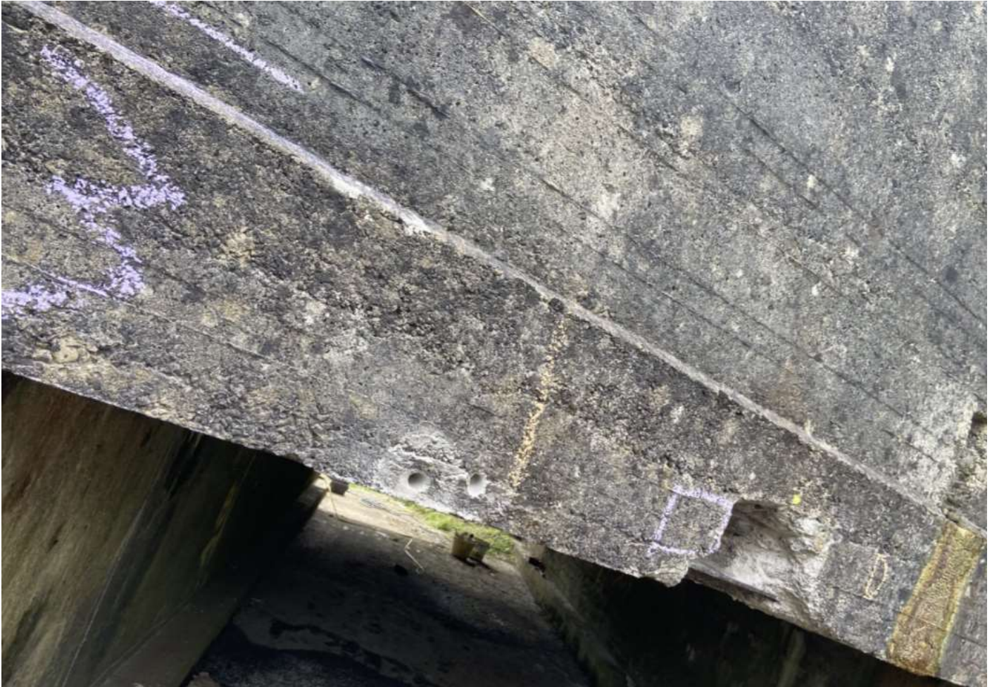
Figure 21: Wide angle view of test area including drill holes for dust samples
