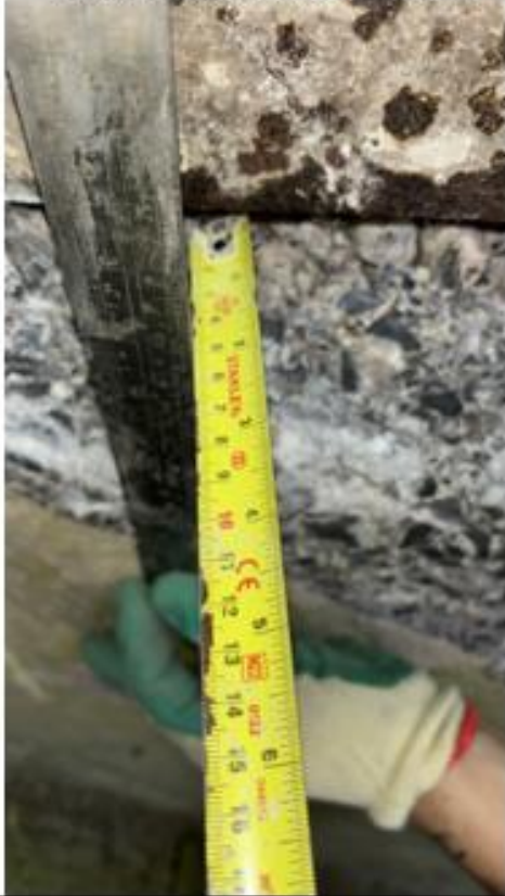
Transverse square rebar cover 51mm
