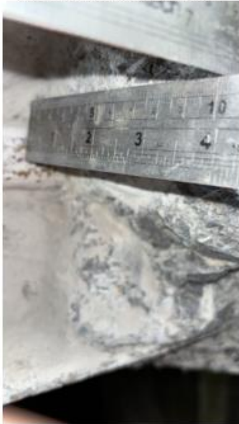
Area 4 –top side flange cover 104mm
