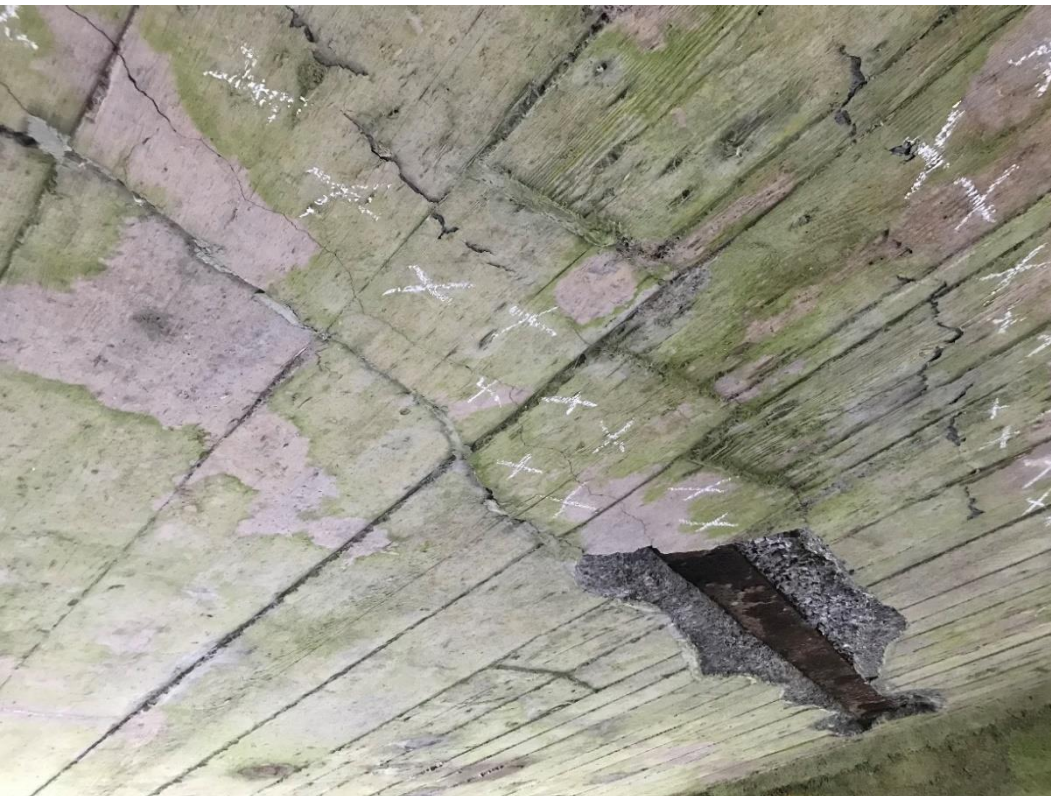
Figure H-20 – North span - exposed filler beam with delamination evident
