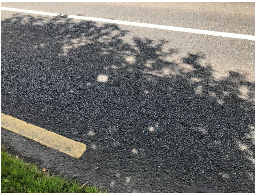
Figure H-2 - View of the cracking to the northwest corner of the carriageway
