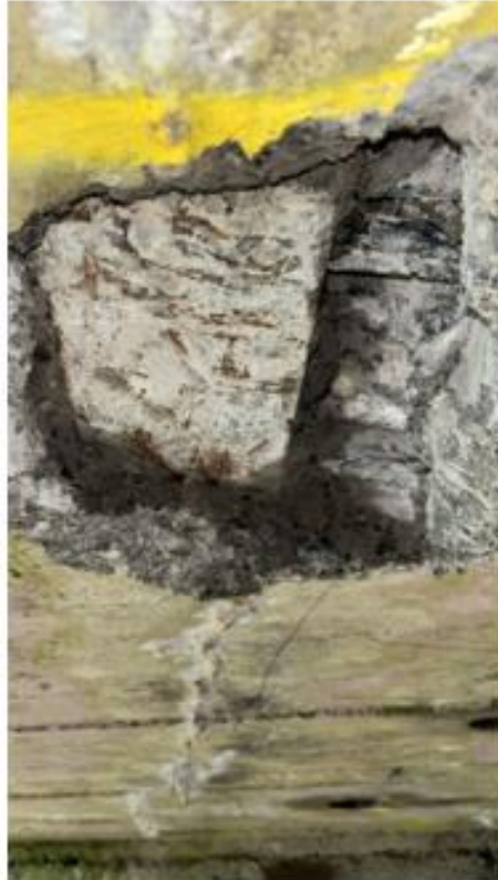
Area 3.1 Soffit breakout
