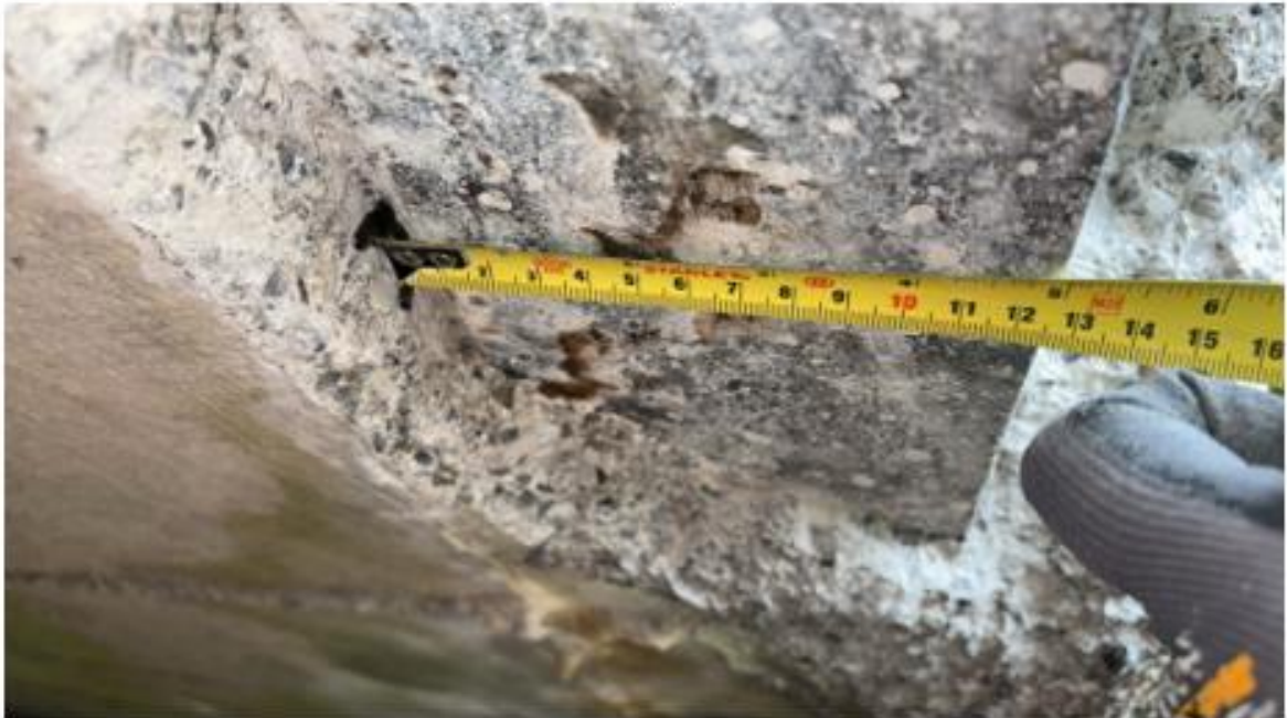
Area 3 - Bottom flange 124mm width
