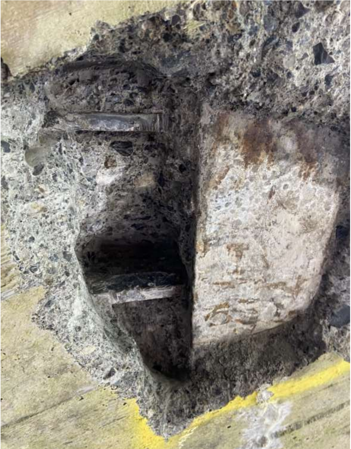
Figure 27: Longitudinal cover was 39mm, Transverse cover was 54mm
