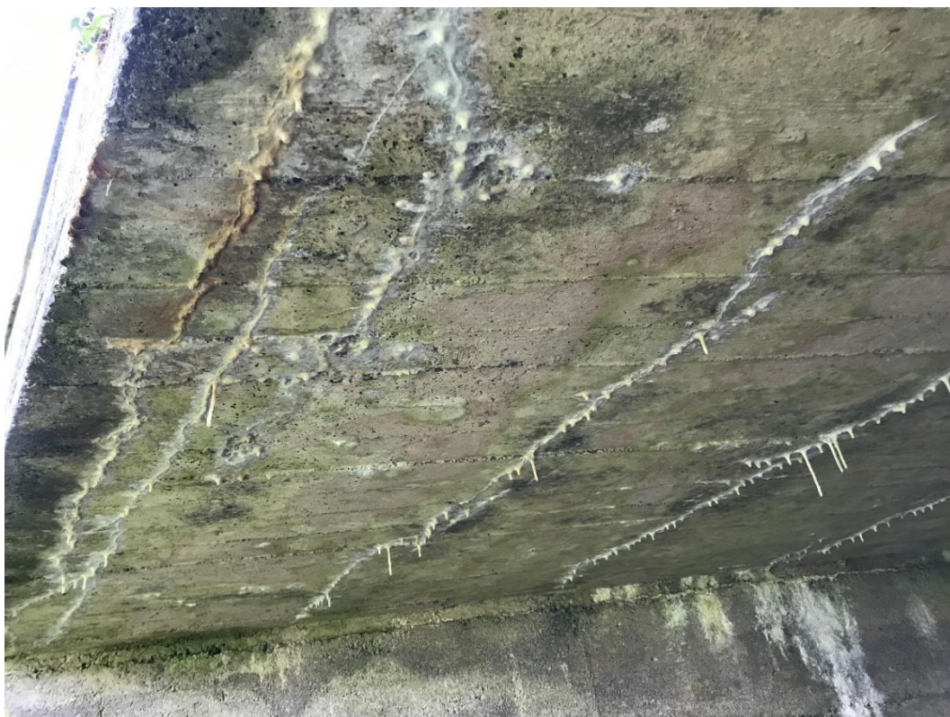
Figure H-17 - South span - Cracking sealed with calcite
