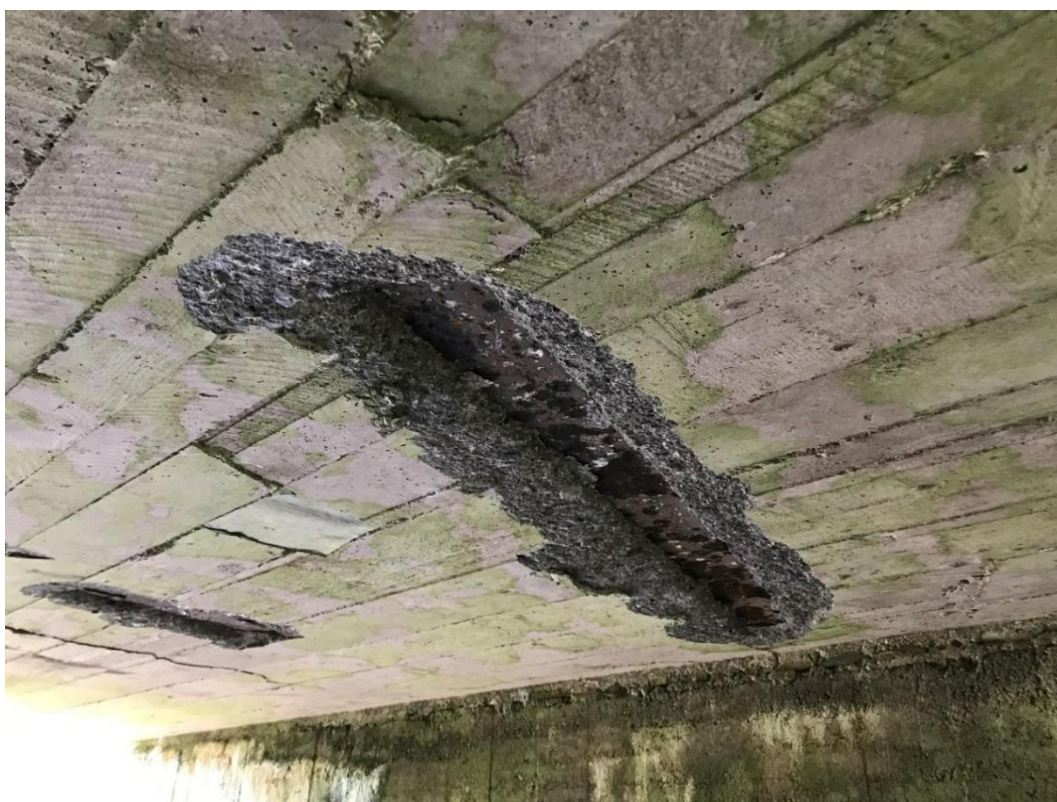
Figure H-18 - South span - spalling with exposed filler beam
