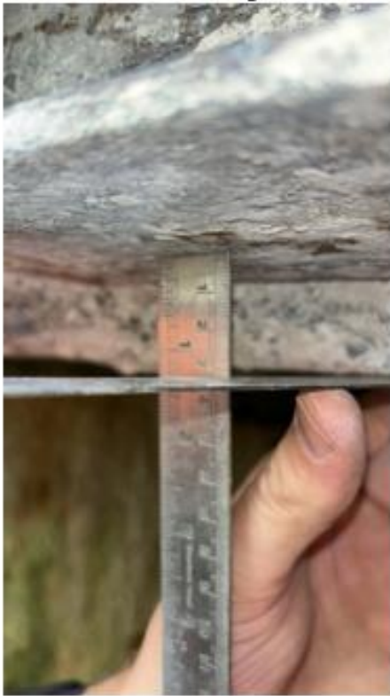
Area 3 - Top side flange 105mm cover side
