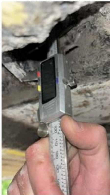
Transverse rebar 28.9mm
