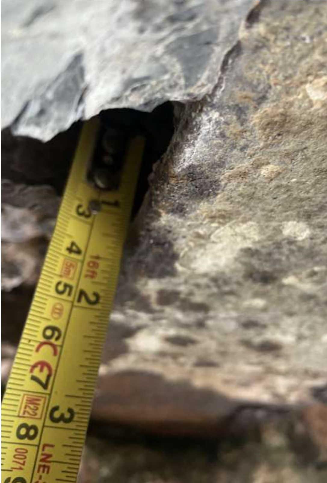
Figure 41: Cover of Transverse steel
