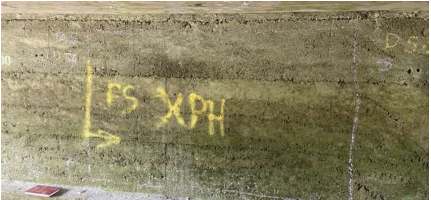
Figure 44: Pilot hole reinstatement along with dust sample holes
