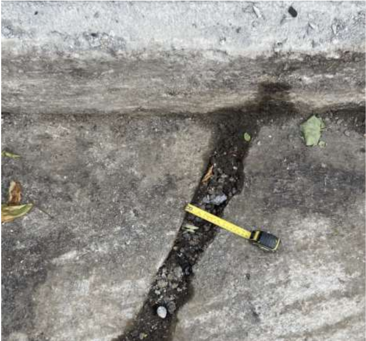
Figure 19: 90mm cutout in deck surface
