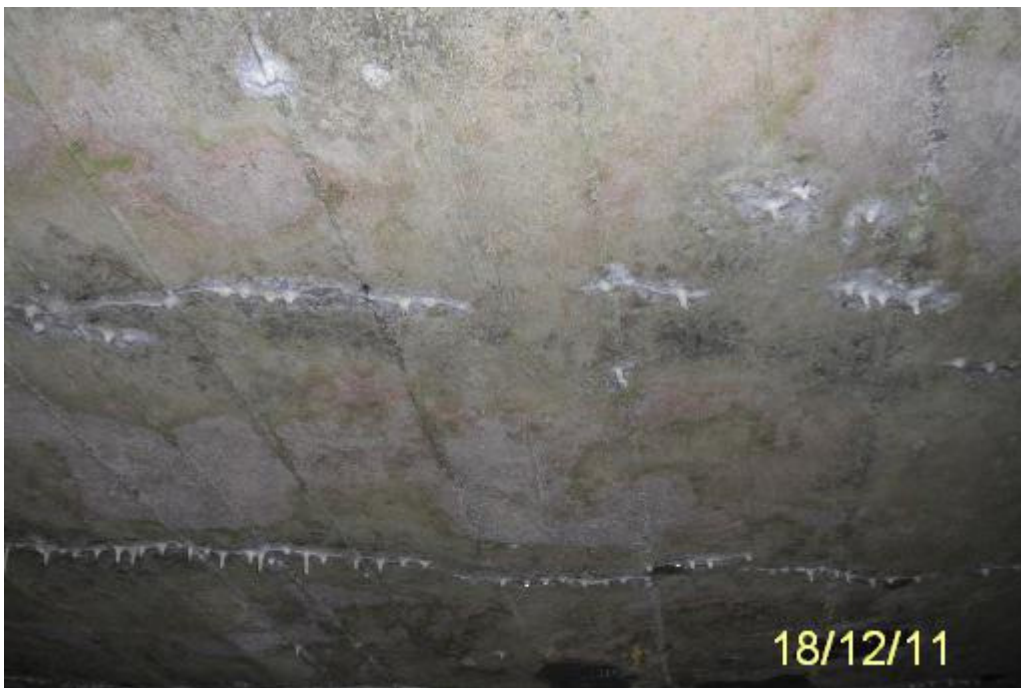
Photo 10. Span 1 soffit – water seepage & calcite staining
