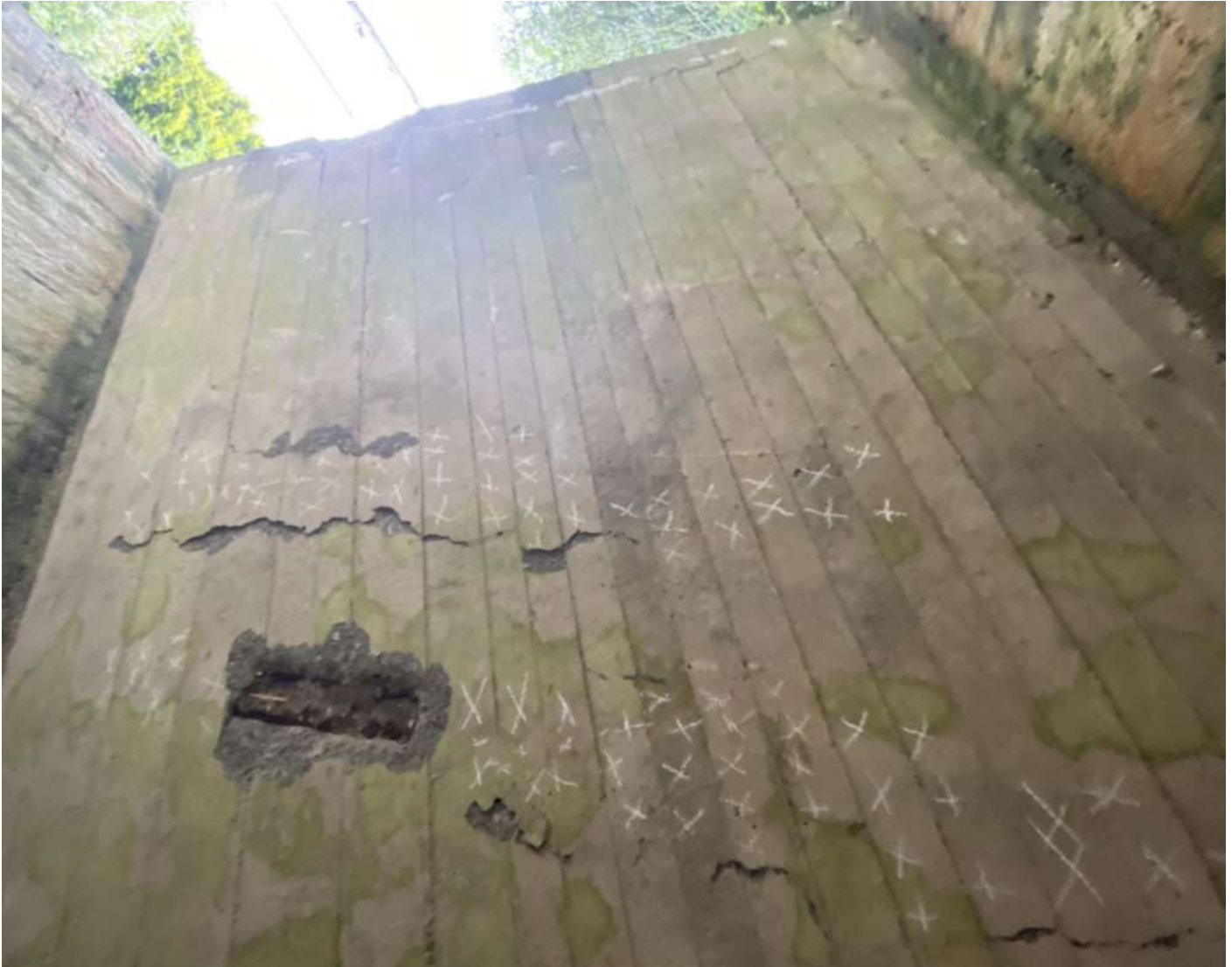
Figure 31: Delamination denoted by white x chalk marks
