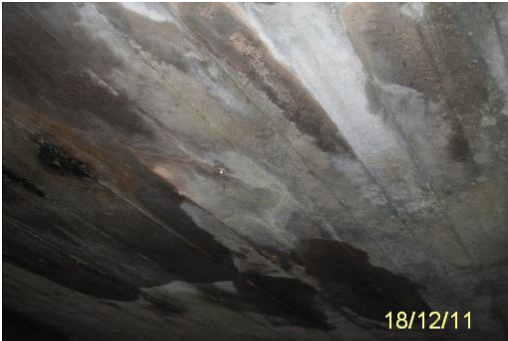
Photo 11. Span 2 soffit – water seepage
