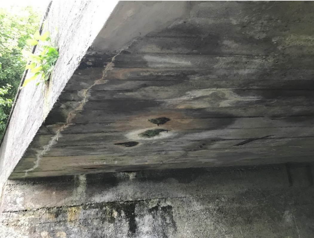
Figure H-19 - North span - cracking sealed with calcite, water staining and spalling
