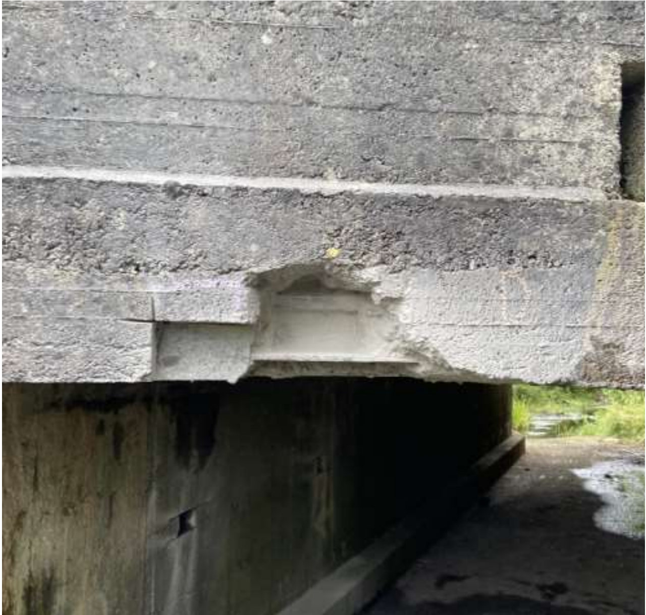
Figure 23: Carbonation test sample extracted to the left of breakout
