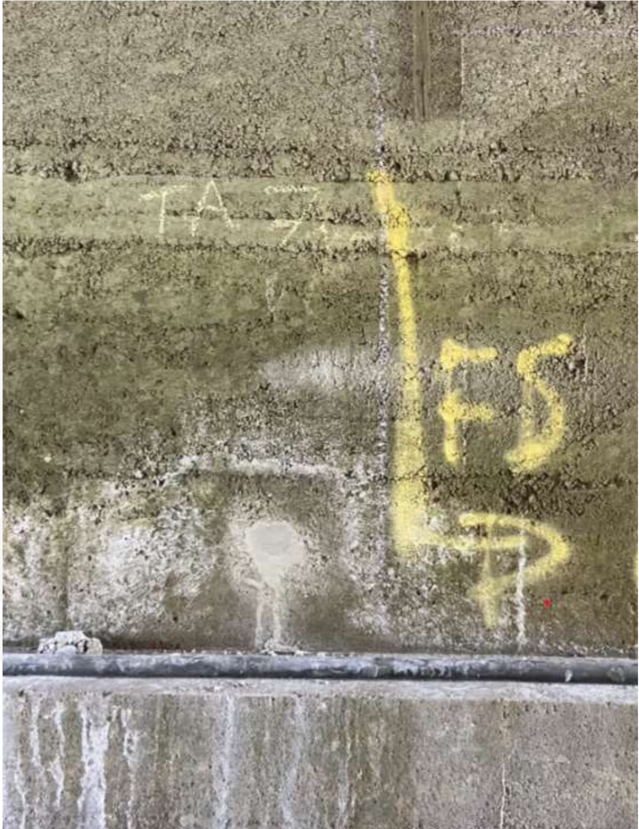
Figure 51: Pilot hole reinstatement
